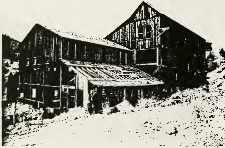
Figure 152. Arsenic plant (structure #59), northwest view.
